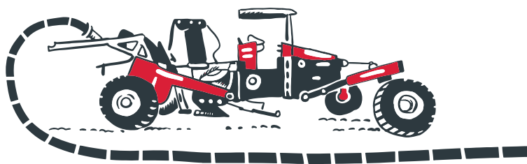
Laying chute 2x 20 kV plowing in of 2 x 20 kV medium-voltage systems
